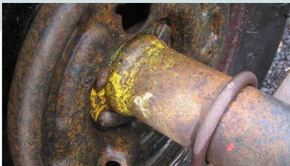
Yellow paint dab typical 68-70 staggered shock housings
