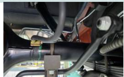
Staggered shock installation
