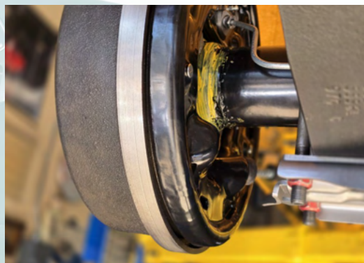
Incorrect installation and fit
